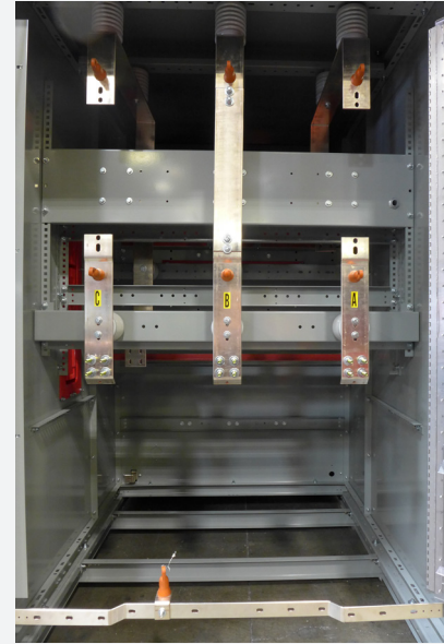
Utility Compartment Main Bus
