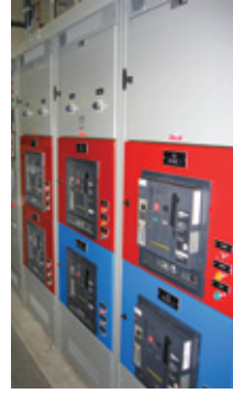
Compartment doors were specified to be color coded for ease of identification during any power system problem
