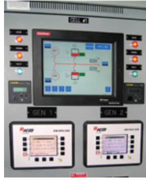
IEM Canada EASYGEN 3200 Series engine controllers and GE Fanuc 90-30 series PLC for Master Controls
