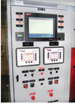
IEM Canada EASYGEN 3200 Series engine controllers and GE Fanuc 90-30 series PLC for Master Controls
