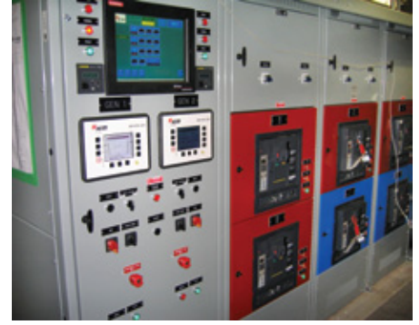
Compartment doors were specified to be color coded for ease of identification during any power system problem
